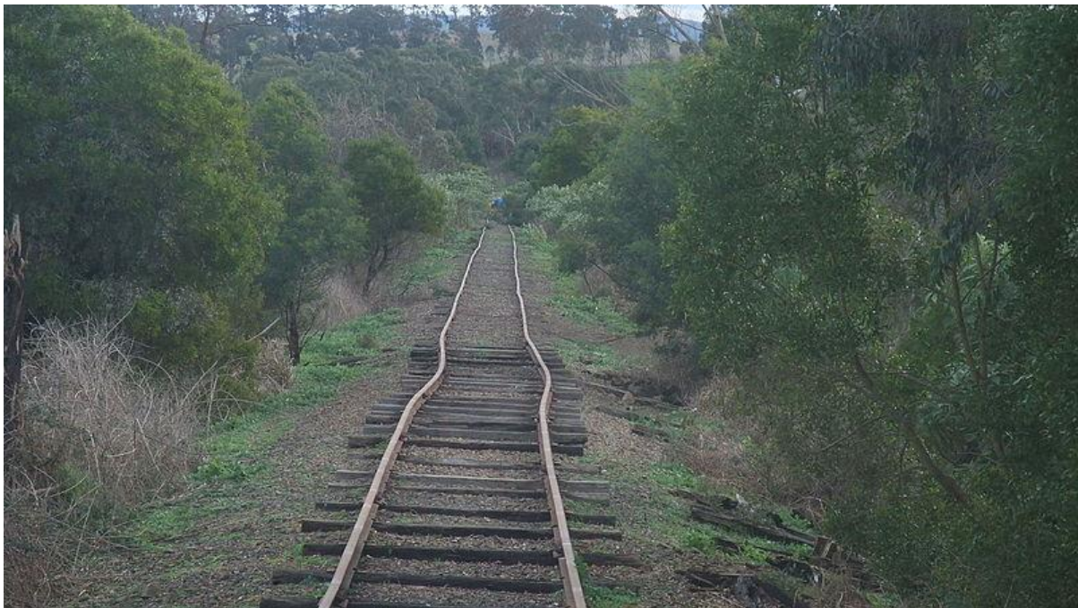
Figure 9-1 Thermal buckling of railway tracks
